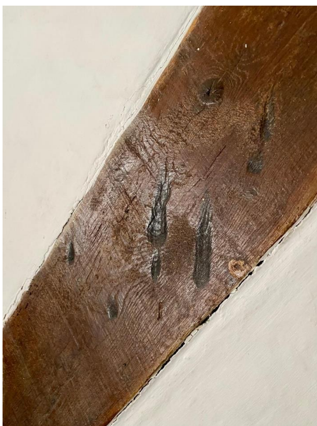
1 st floor bedroom south of chimney stack = 9 burn marks., mainly around fire place.
